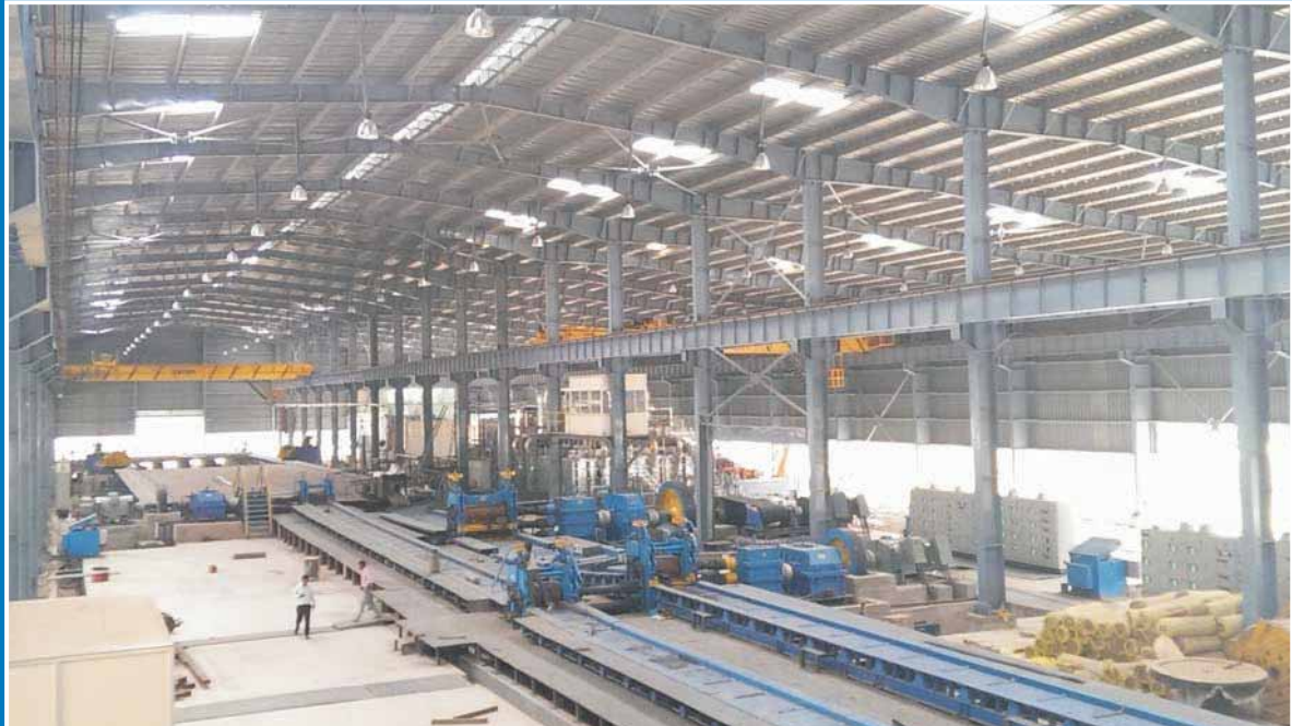
Interior view of the Steel Rolling Mill of the Company at Alwar, Rajasthan.
